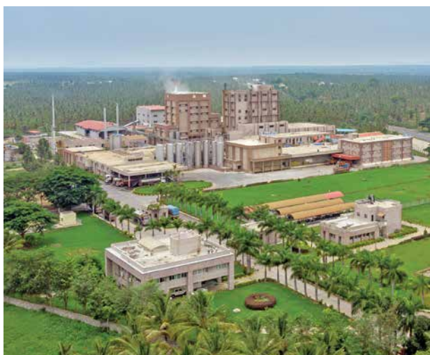
Nandini Dairy Plant, Channarayana, Karnataka
